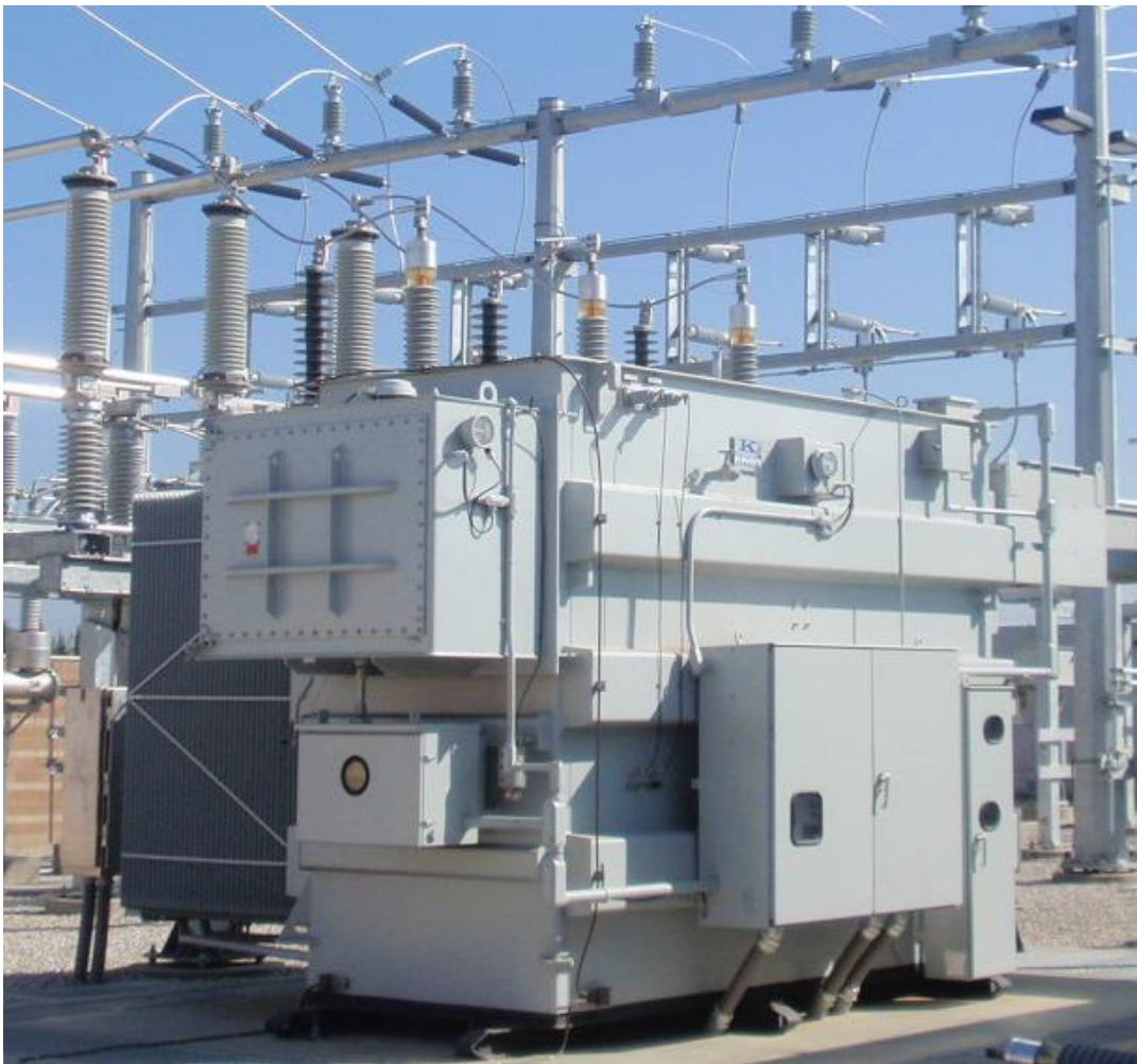
Typical Substation Power Transformer
