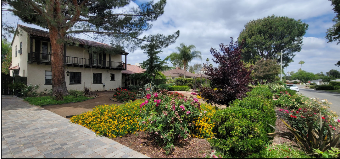
Northeast (Front) Elevation and front yard
