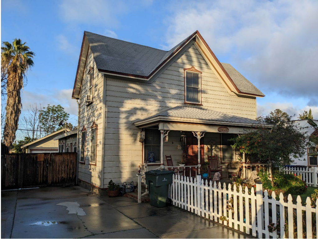
Figure 1 - Front (northeast) elevation, looking west
