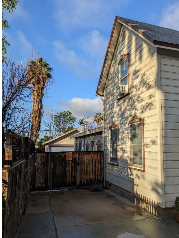
Figure 3 - Side (southeast) elevation, looking west
