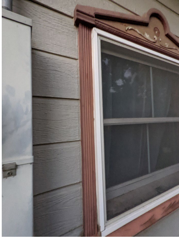
Figure 5 - Detail Photo showing modern siding, modern side window trim, and clad windows
