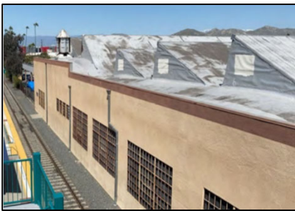
Plant 1 West Elevation, Looking Northeast; 2021
