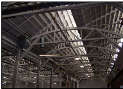
Plant 1, Bowstring Truss and Sawtooth Roof Looking West/Southwest; May 2007
