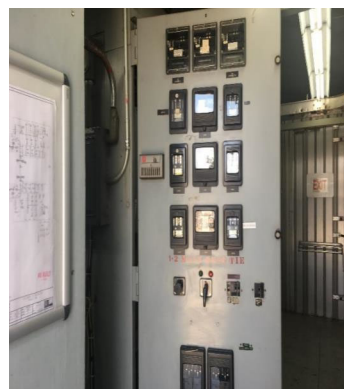
Typical Electromechanical Relays
