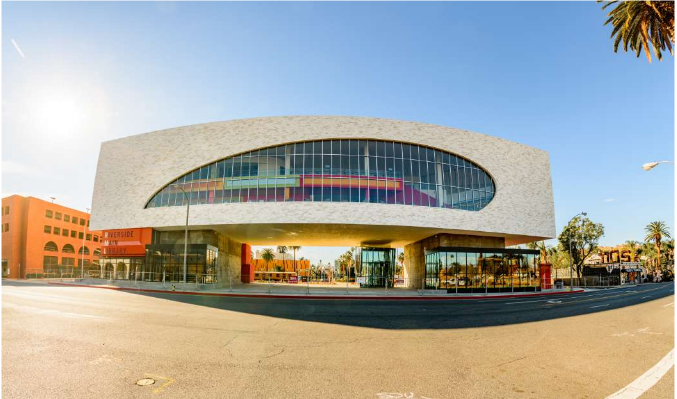
Figure 4.3.9 Main Library Facing Mission Inn Ave
