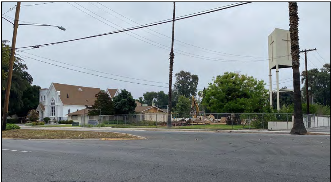
Magnolia Presbyterian 1965 Sanctuary Demolition May 2021
