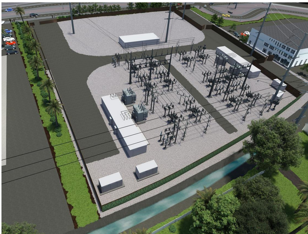
Proposed Low Profile Hunter Substation Replacement
