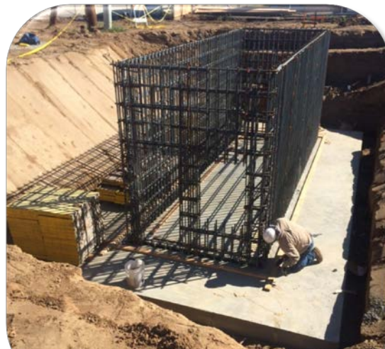
Plaza Substation Power Pit Construction (MPRP Project)
