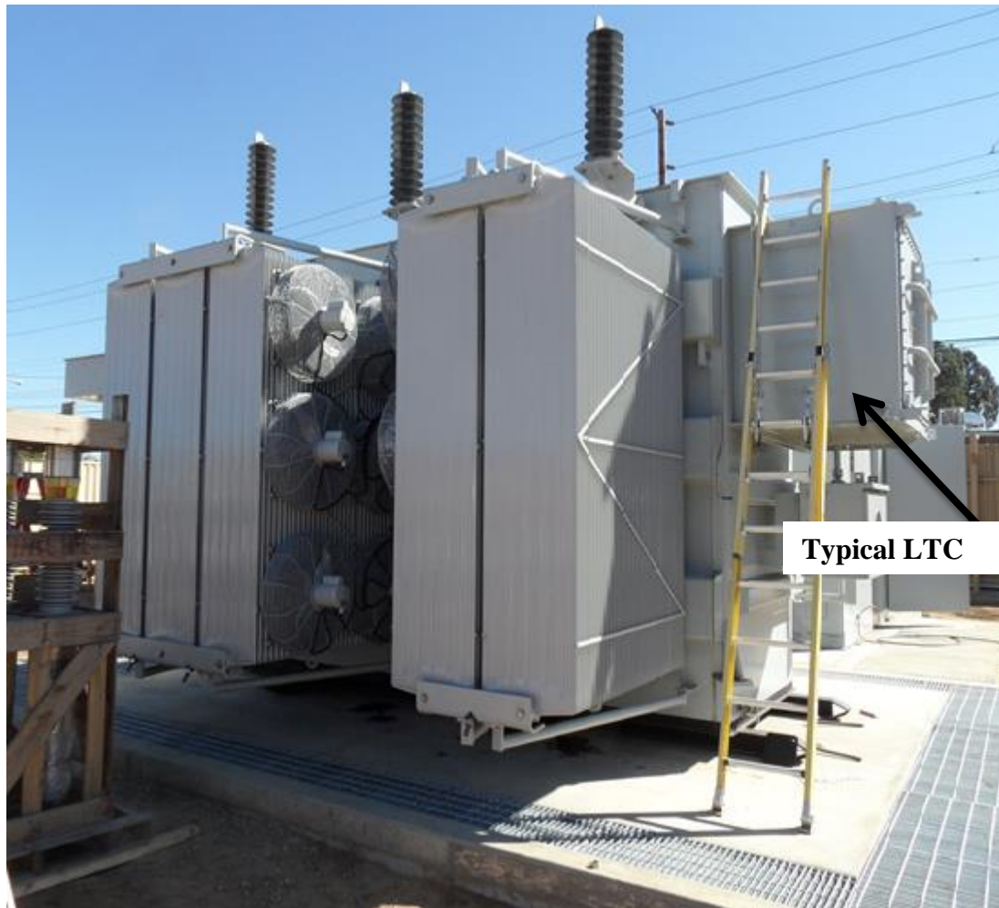
Typical substation transformer with Load Tap Changer (LTC)
