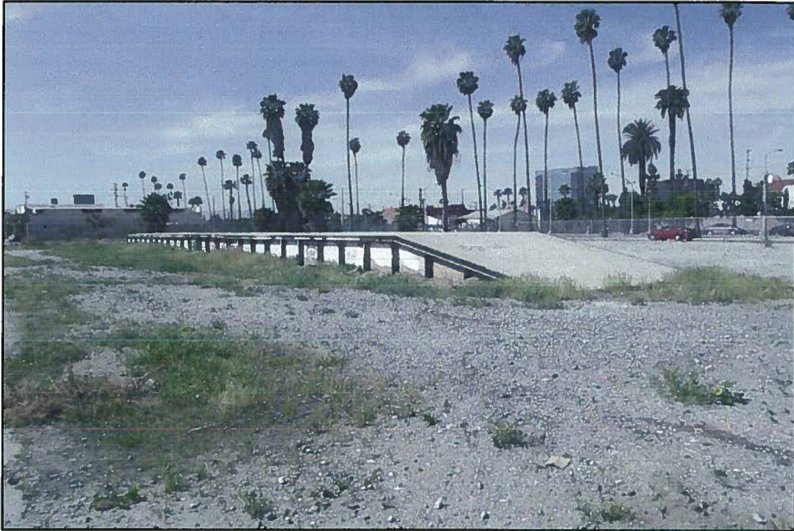
Figure 11. SPRR Loading Platform Framed with Scrap Railroad Track
