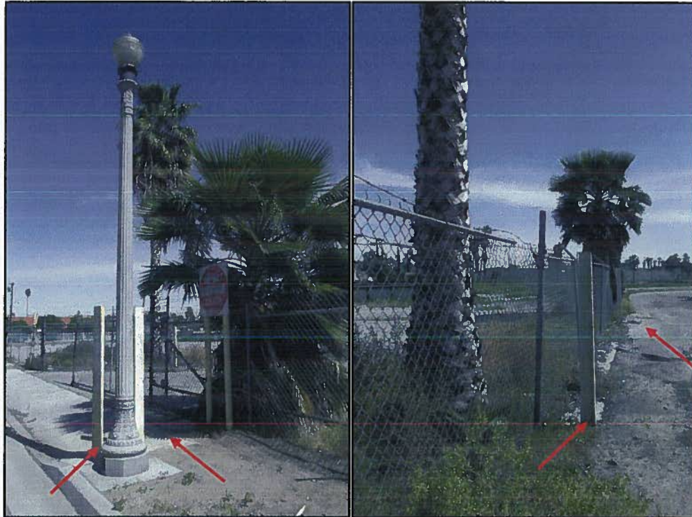
Figure 14. Former SPRR Track in Use as Bollard Posts
