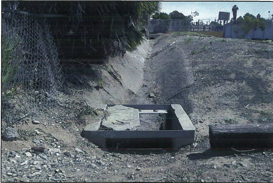
Figure 4. Brow Drainage Ditch (ca. 1960) in the Project Area
