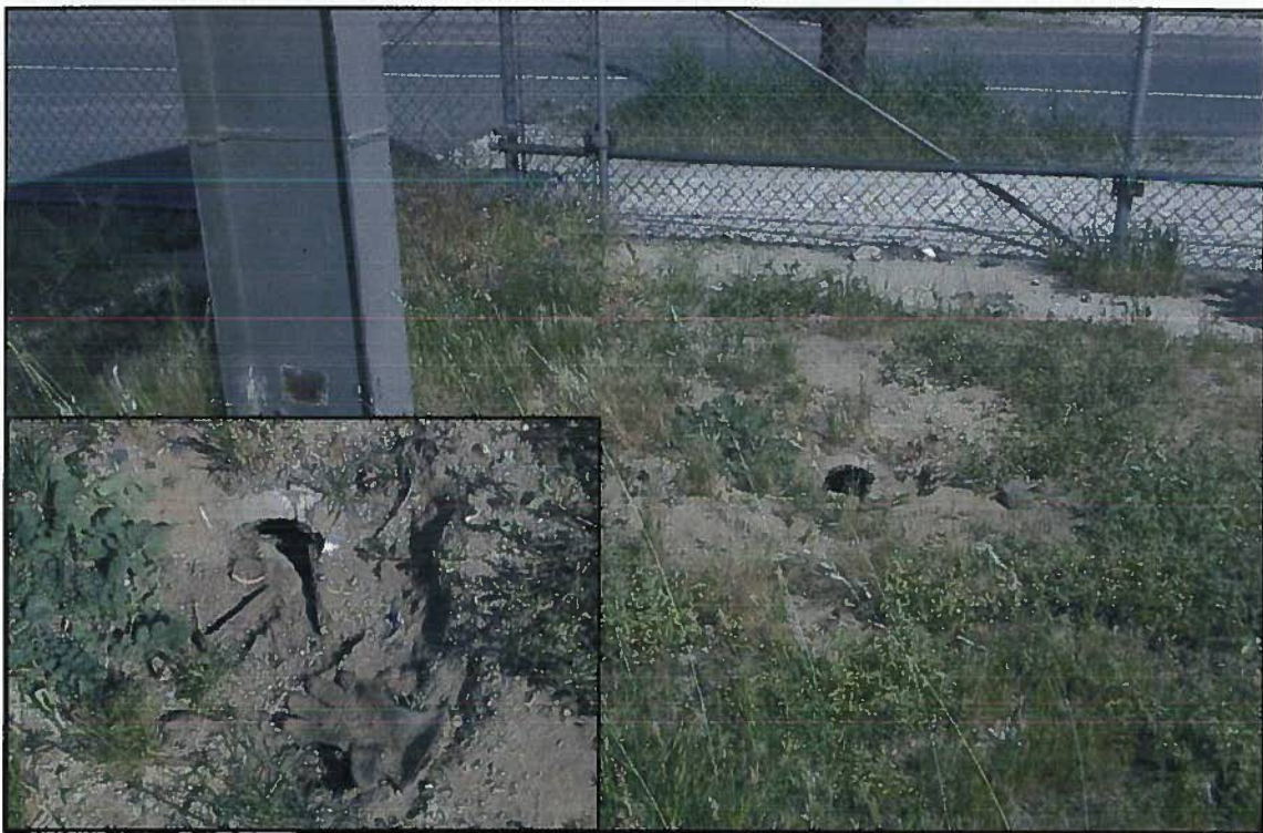
Figure 6. Broken Clay Sewer Pipe within Project Area
