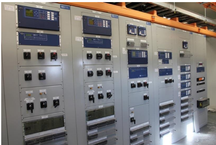
Typical Substation Protection Panels
