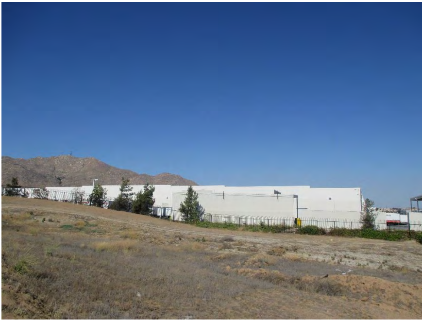
Buildings to the east
