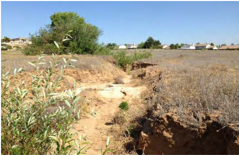
Drainages feature looking northwest
