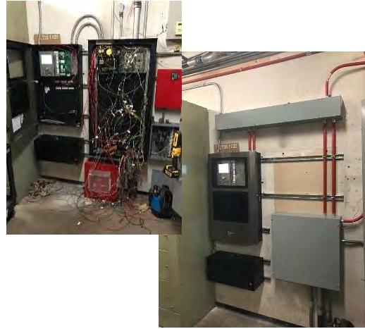
Fire Life Safety System Panel Replacement
