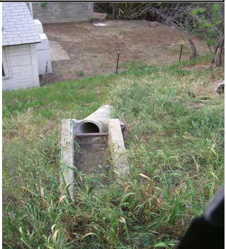
FIGURE 77: IRRIGATION WEIR BOX AND PIPE
