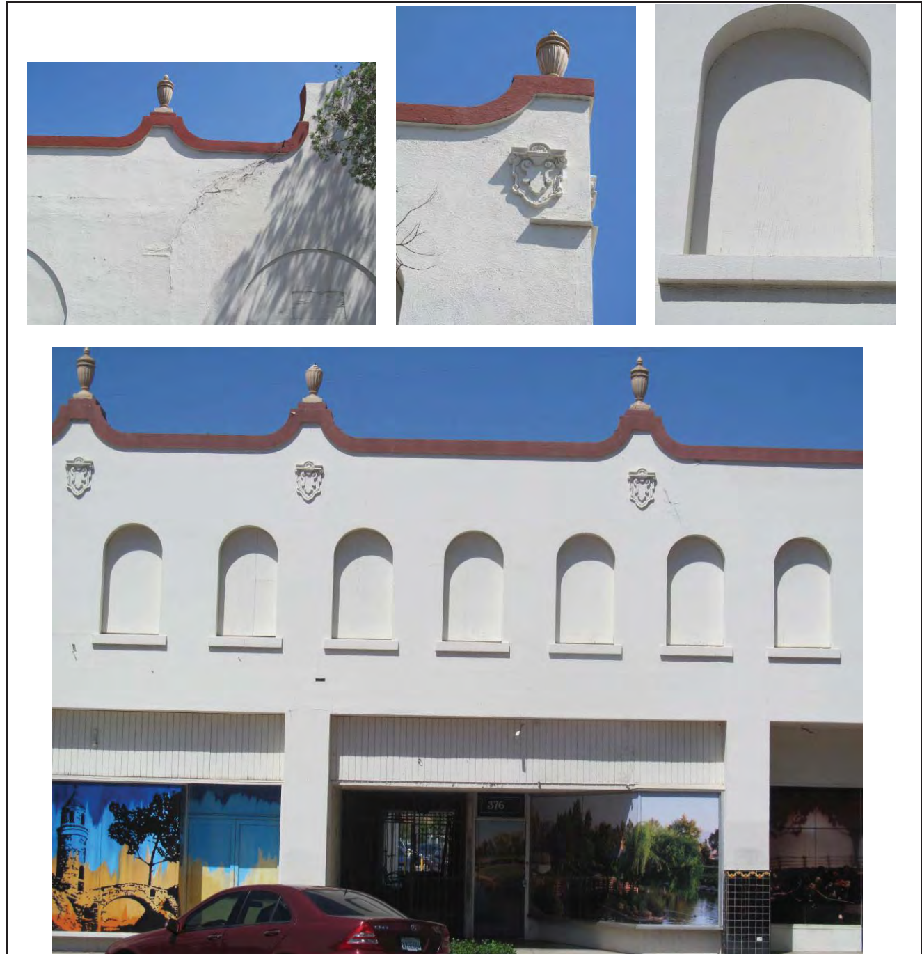
GTL | MHA, August 2016 site recordation photograph; Detail views of various terra cotta urn, parapet and cartouche conditions, south and west façade. Station point is from street.
