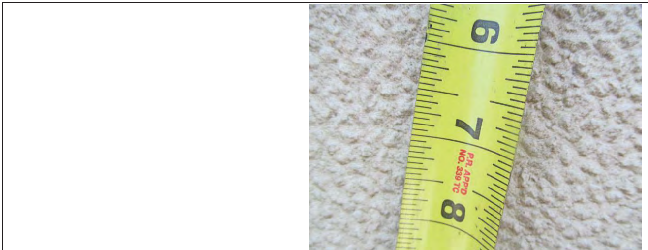
GTL | MHA, August 2016 site recordation photograph; Detail view of second floor glazing: "pebbled" translucent finish.
