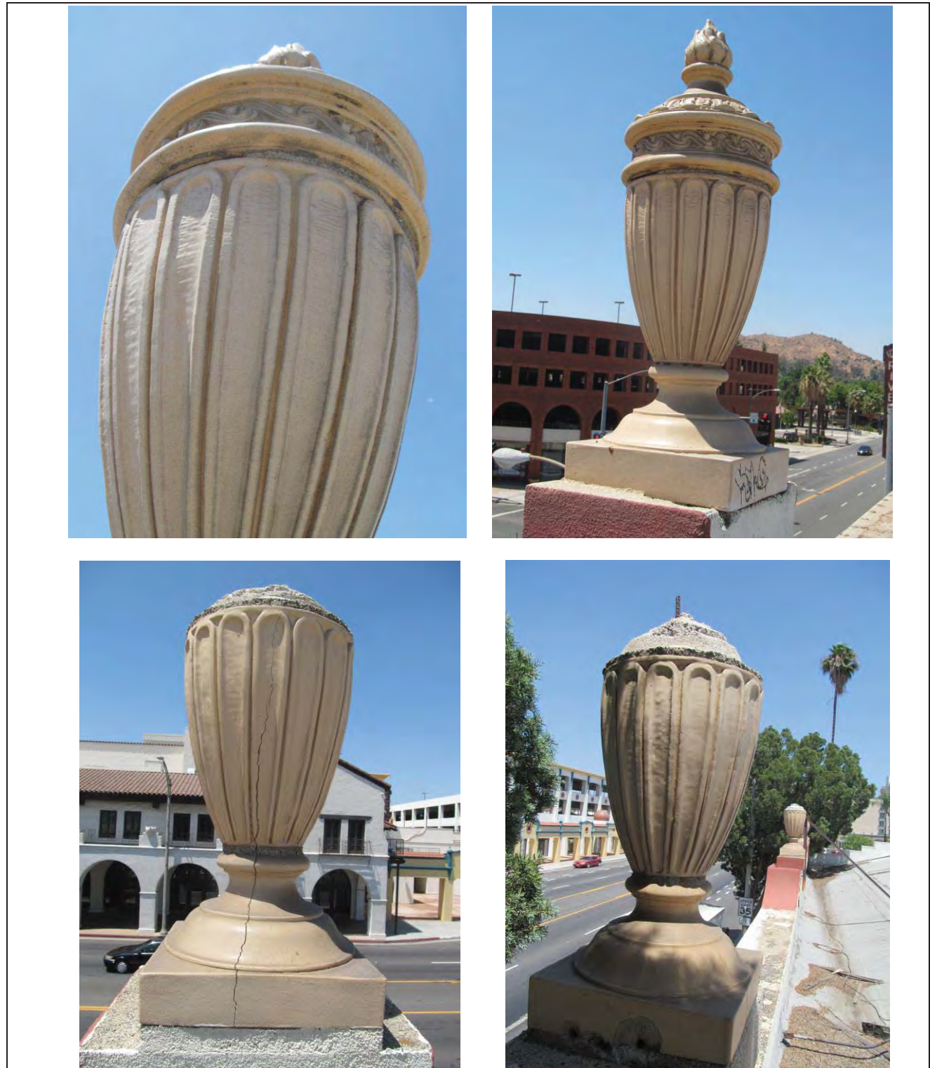
GTL | MHA, August 2016 site recordation photograph; Detail views of various terra cotta urns. Station point is from roof. Note color, finish and texture at fronds; construction in three-piece casts, cemented together around a single .5" square reinforcing steel rod, and consequent longitudinal cracking.
