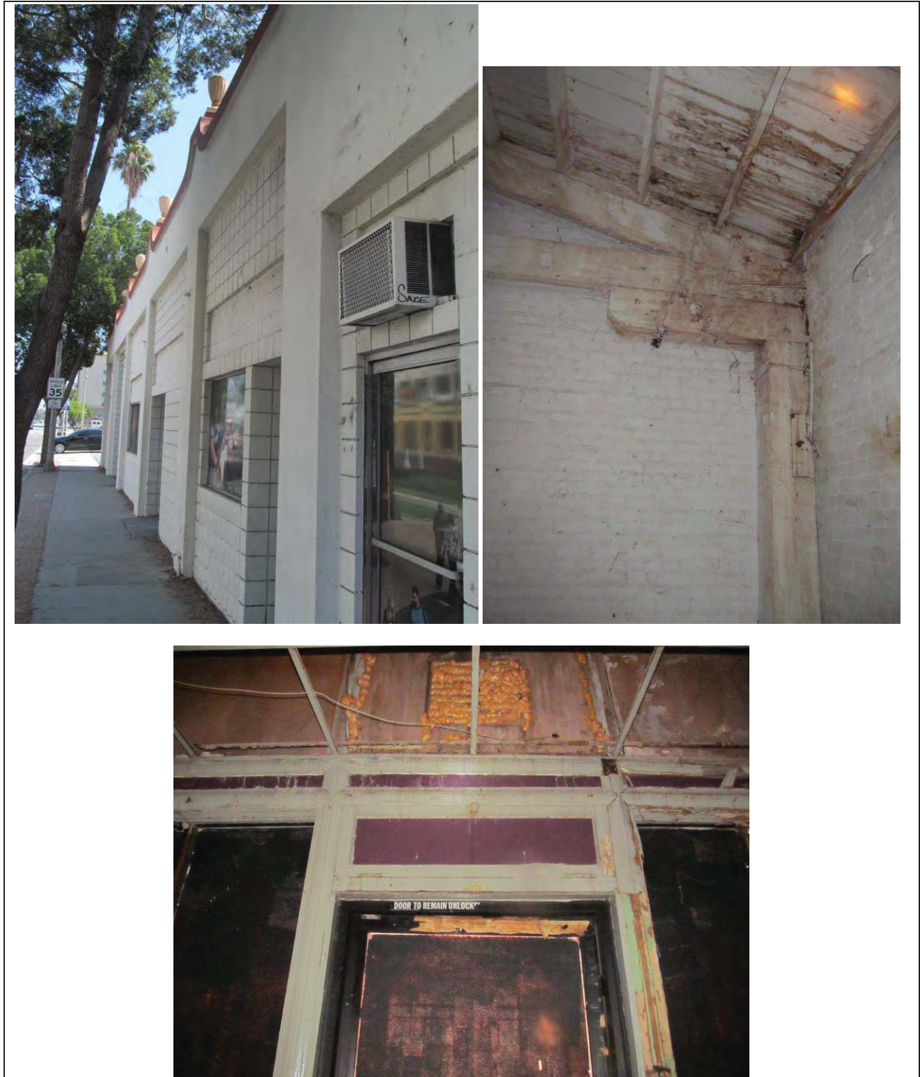
GTL | MHA, August 2016 site recordation photograph; Detail view of west façade existing storefront not dated from significant era, and presumed original G. Stanley Wilson storefront, exposed interior view & detail. Wood truss at north interior wall.
