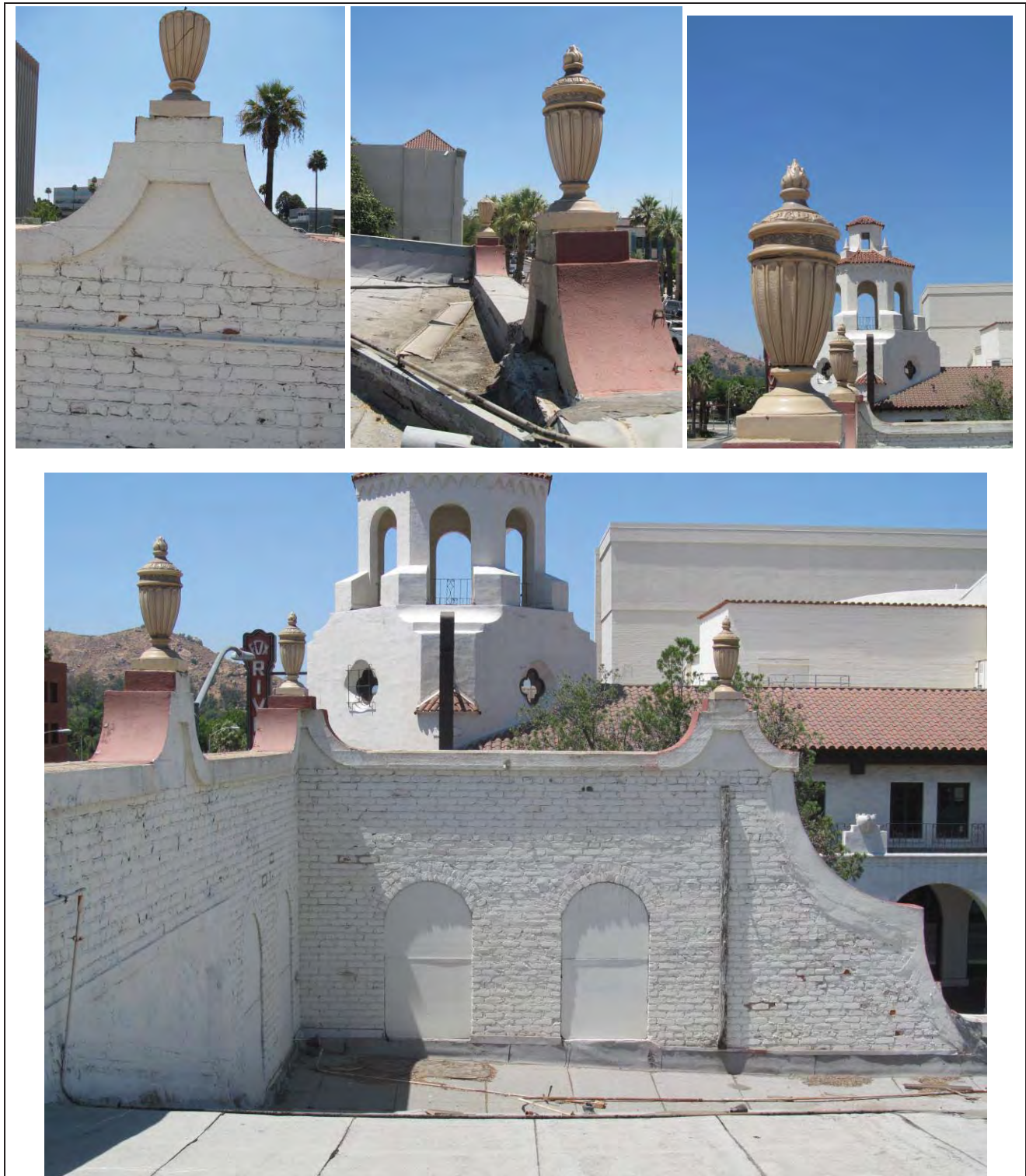
GTL | MHA, August 2016 site recordation photograph; Detail views of various terra cotta urn & parapet condition Station point is from roof, view west. Note covered window openings and drop in façade. Tower beyond is Fox Theater.
