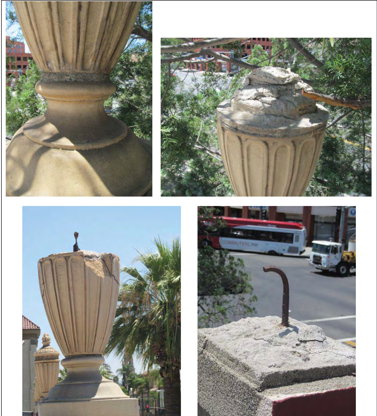
GTL | MHA, August 2016 site recordation photograph; Detail views of various terra cotta urns. Station point is from roof. Note color, finish and texture at fronds and base; construction in three-piece casts, cemented together around a single .5" square reinforcing steel rod, and setting base.
