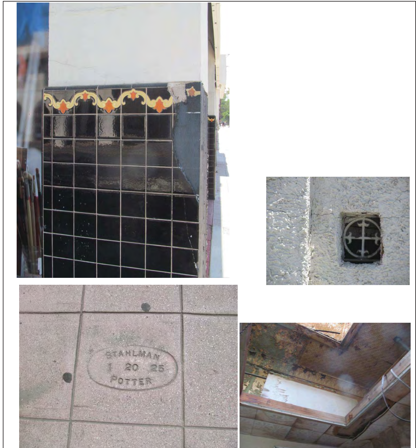
GTL | MHA, August 2016 site recordation images: Detail view of sidewalk paving stamp. Tile wainscot not considered significant. Cast attic vent at east façade to be relocated in new construction. Tin ceilings have potential reuse.
