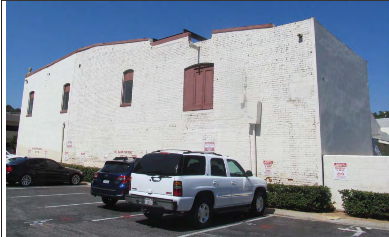
GTL | MHA, August 2016 site recordation photograph; Detail view of east façade remaining of Fire House Number 1. Plastered façade return at left side of image is representative of the extent of the G. Stanley Wilson's façade design modification.
