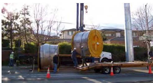
OFFLOADING CABLE REELS AT JOB SITE
