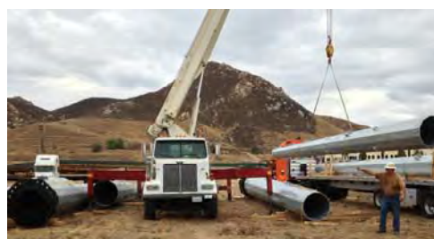
OFFLOADING STEEL POLES
