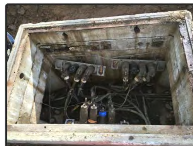
Replacement of antiquated underground cable & devices
