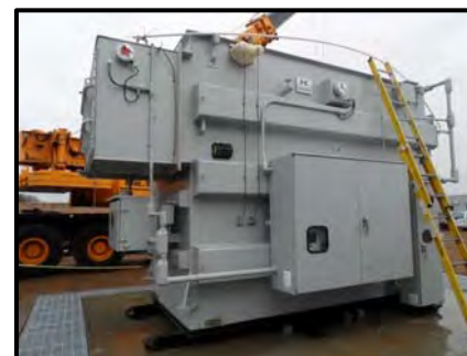
Substation 69-12kV Power Transformer
