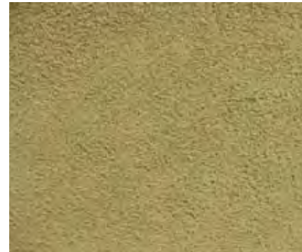
PL-1 LIGHT SAND FLOAT PLASTER - PAINTED (PT-6)
