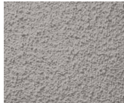
PL-2 HEAVY MACHINE DASH PLASTER - PAINTED (PT-3)
