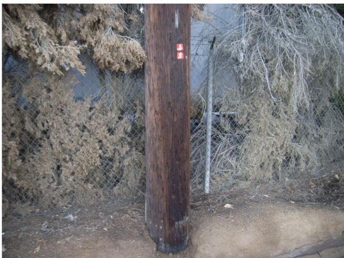
POLE TAGGED FOR REPLACEMENT
