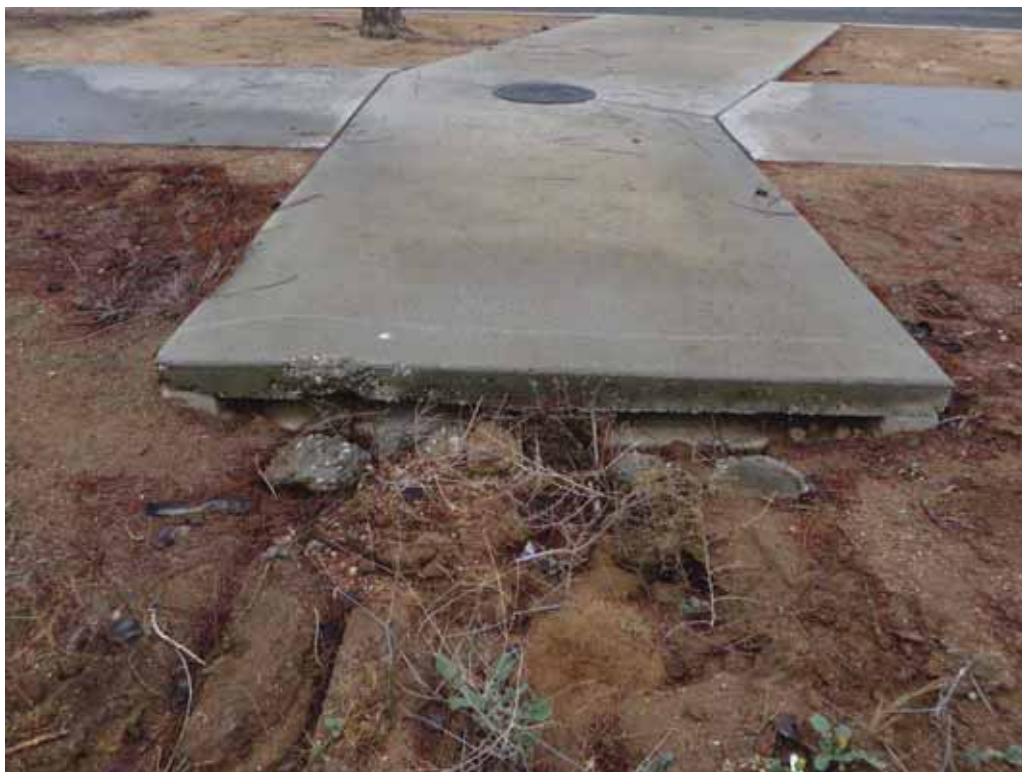
Photograph 10: Concrete inlet structure that receives water from the project site, before flowing into the street gutter and storm drainage system.
