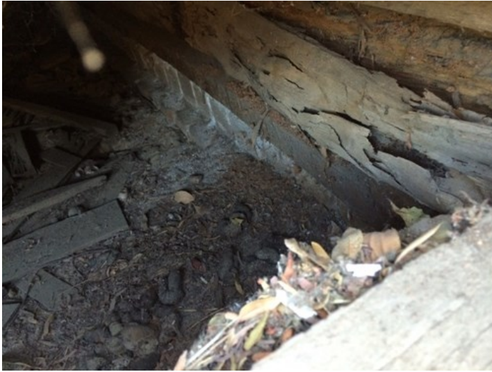
Termite and dry rot damaged floor beam (supports front wall of Harada House)
