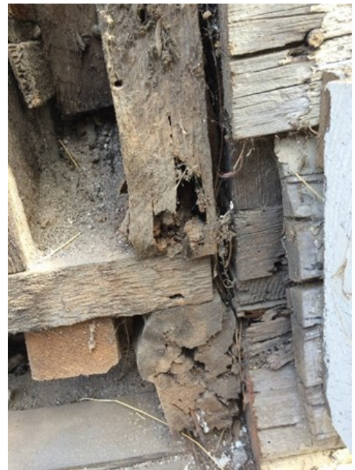
Dry rot damaged floor joist at South Elevation – located at connection of dining room and kitchen
