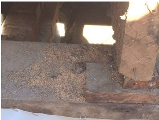
Dry rot damaged floor joist, South Elevation
