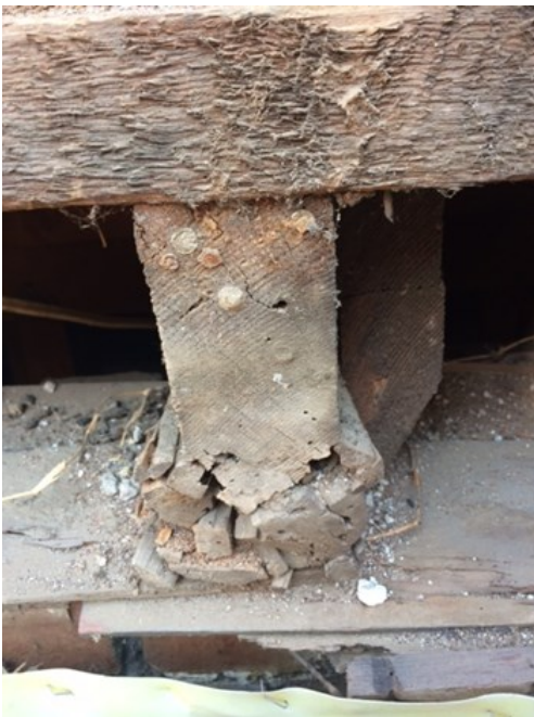
Dry rot damaged floor joist, South Elevation
