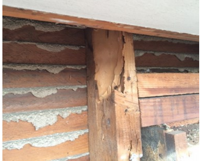
Termite damaged stud at window header, East Elevation
