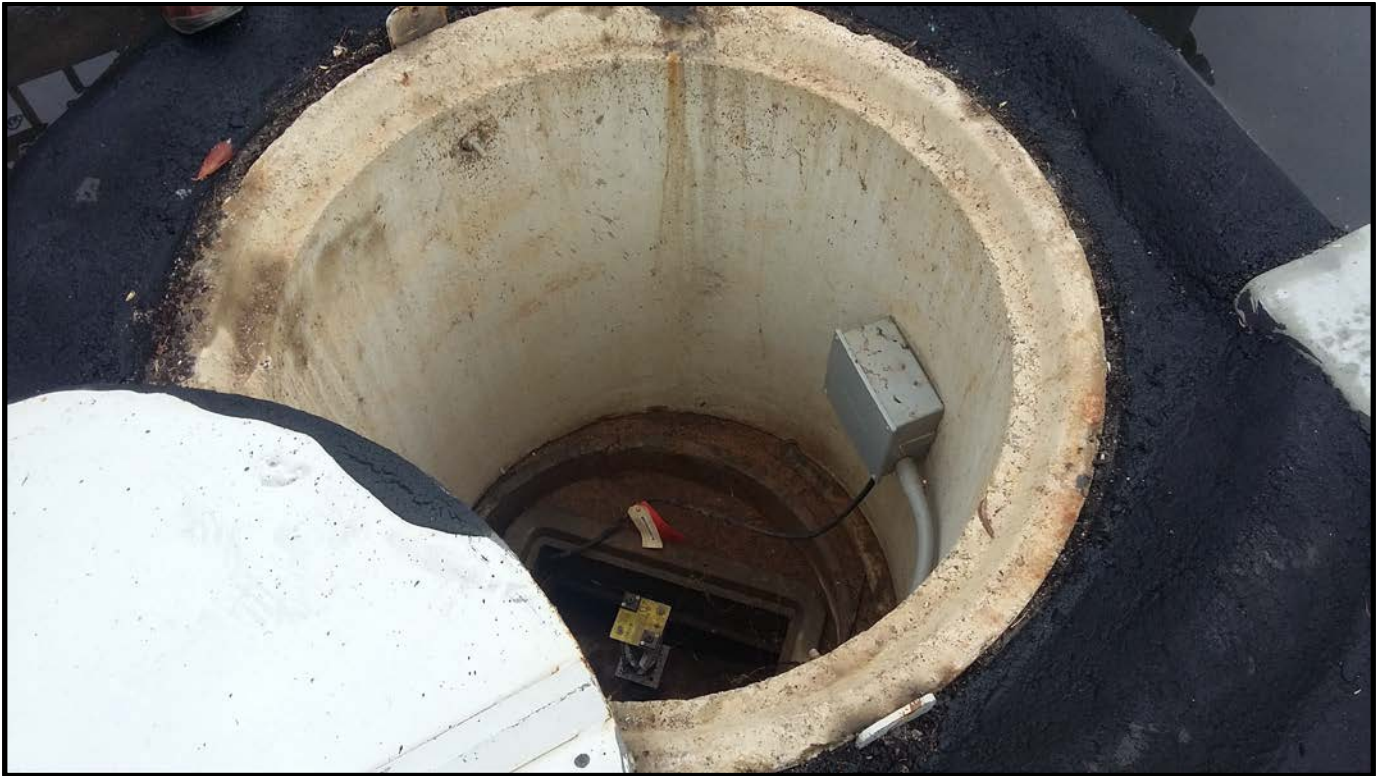
Figure 1 – Existing Circular Vault and Meter at the Mockingbird Canyon Pump Station
