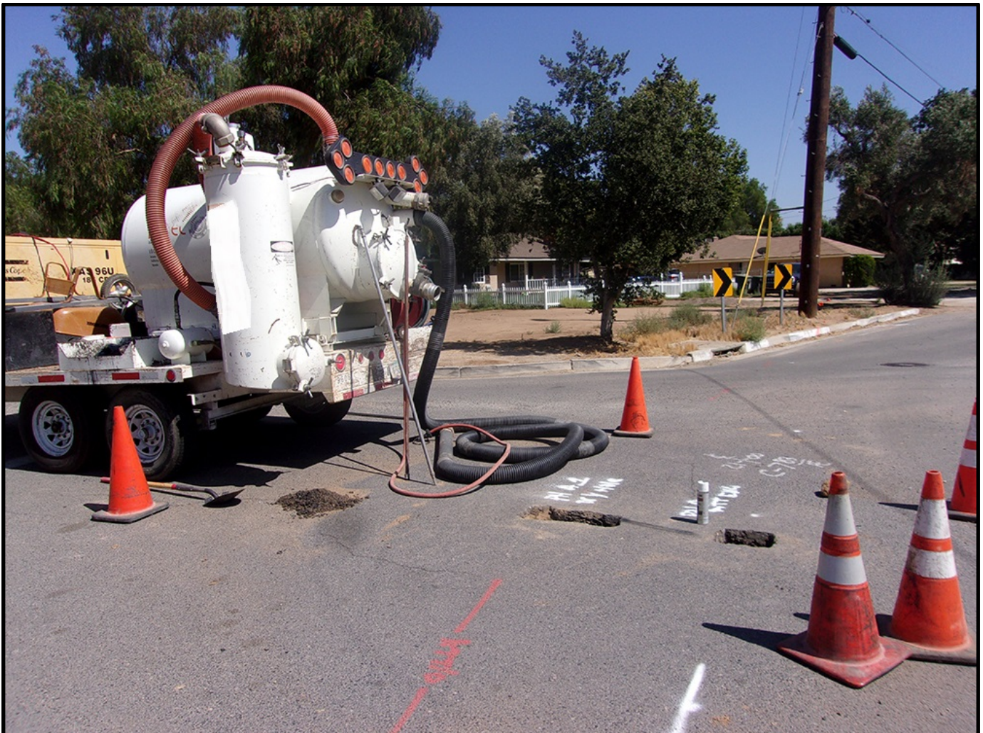
Figure 1 – Typical Utility Potholing Setup for Hydro Excavation with a Vacuum Machine
