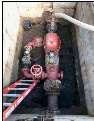
Typical Mechanical Compound Water Meter Installation
