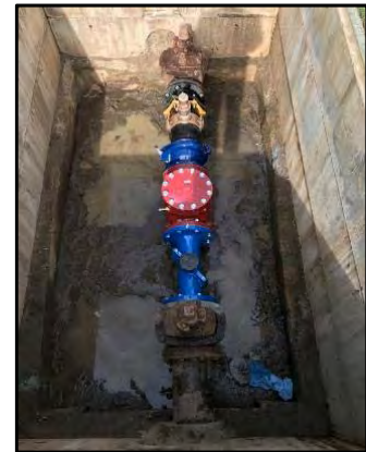
Typical Ultrasonic Water Meter Installation
