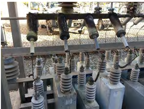
Capacitor Failure at Harvey Lynn Substation
