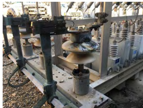
Capacitor Failure at Harvey Lynn Substation
