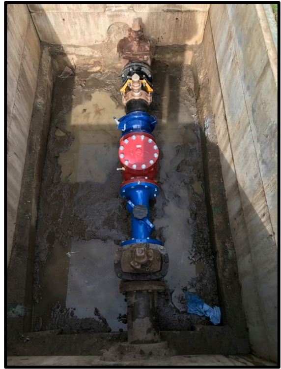
Figure 3 – Typical Ultrasonic Water Meter Installation
