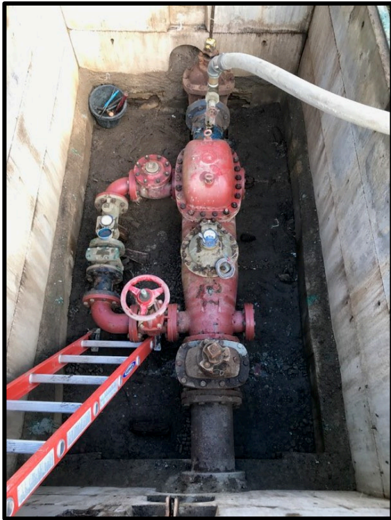
Figure 2 – Typical Mechanical Compound Water Meter Installation
