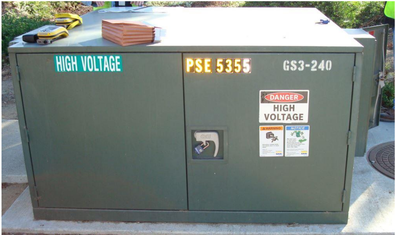
Existing Automatic Transfer Switch
