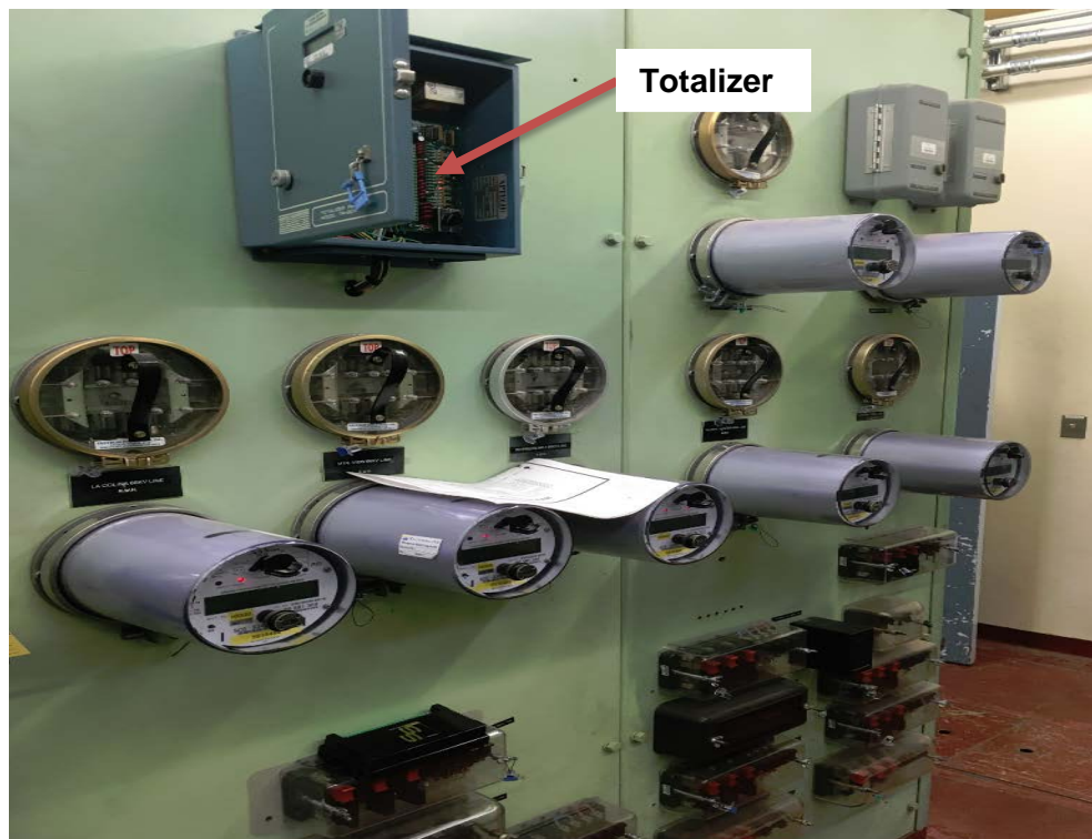
SEVEN (7) CAISO METERS AND TOTALIZER AT SCE VISTA SUBSTATION CONTROL BUILDING
