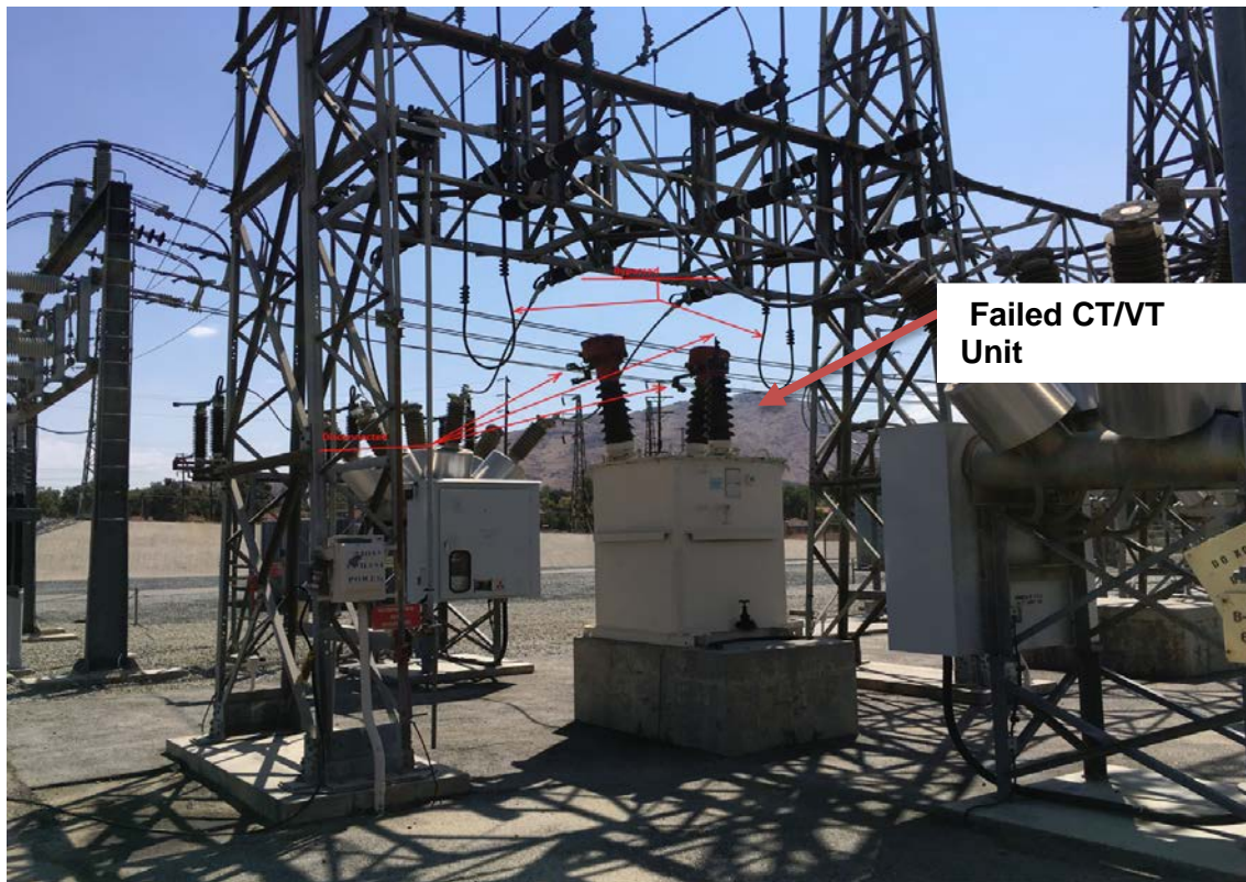
69KV Metering PT – SCE Vista Substation
