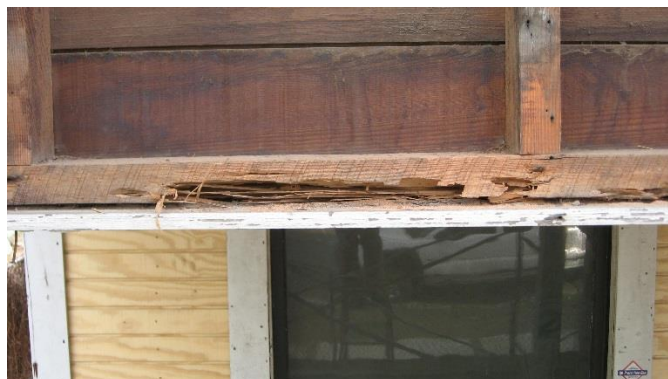
Example of damaged framing requiring emergency repair.
