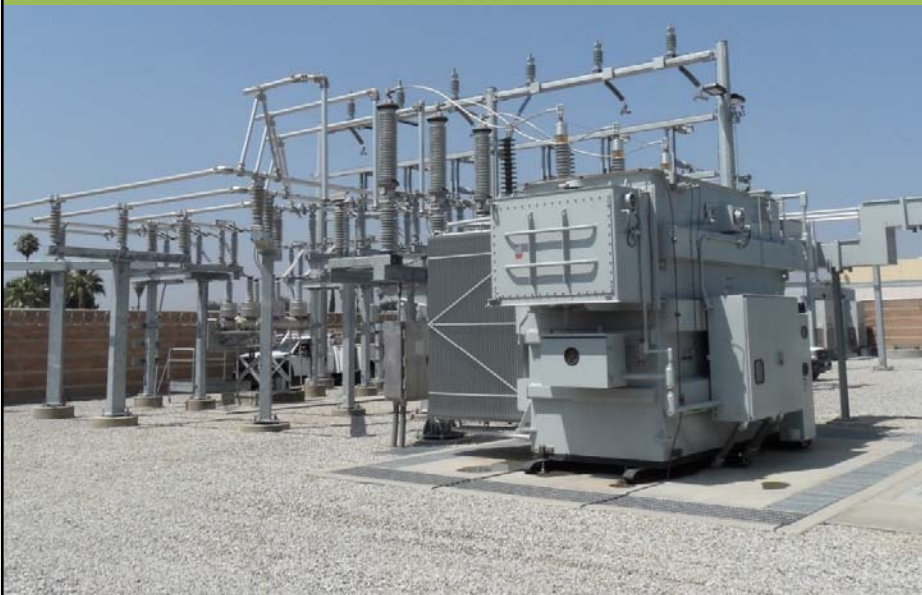
Transformer Addition, Hunter Substation
