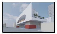
Riverside's proposed main library would be a two-story, 35,000-square-foot, building that would be elevated on a 30-foot pedestal to create a plaza and pedestrian walkway underneath. The outer walls of the rectangular structure would be covered in white marble-look porcelain tile and plaster. An asymmetrical teardrop window would open horizontally onto the warm wood interior. The \$40 million design includes an outdoor terrace at one corner that could
