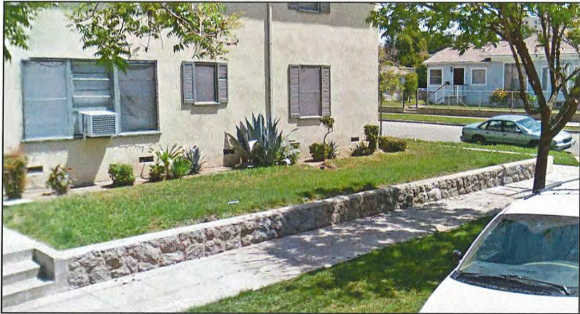
Plate 5.3-1: View of a stone veneer retaining wall at the northwest corner of Chestnut Street and Sixth Street.
