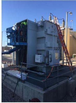
RERC GSU 1&2 Reconditioning
