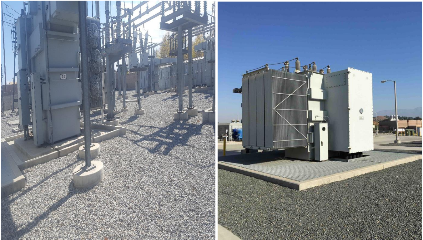
Typical Substation Power Transformer
