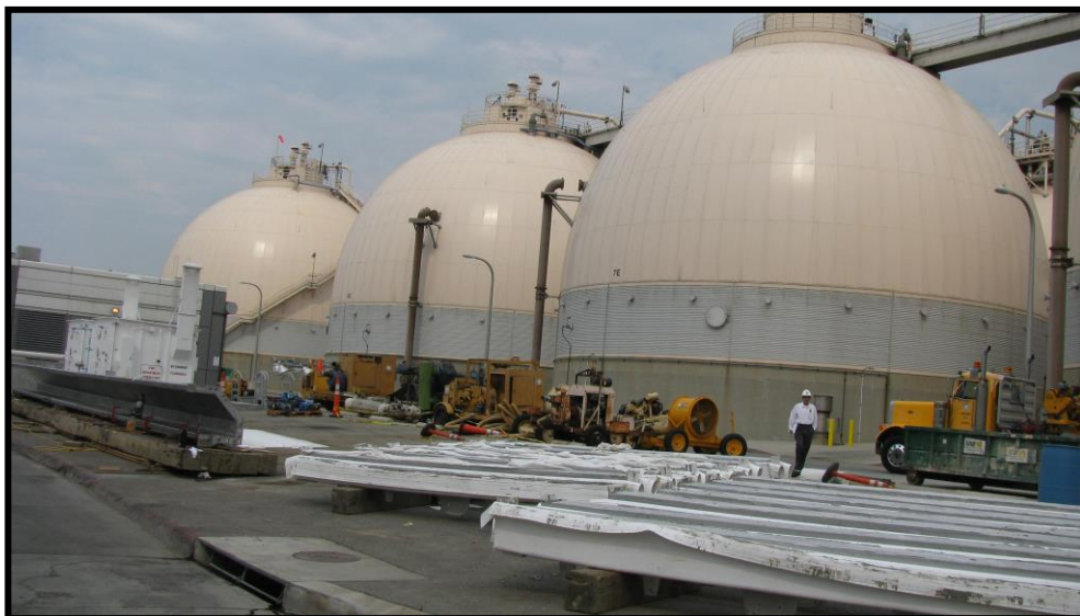
Anaerobic Digesters at Hyperion WRP- City of Los Angeles
