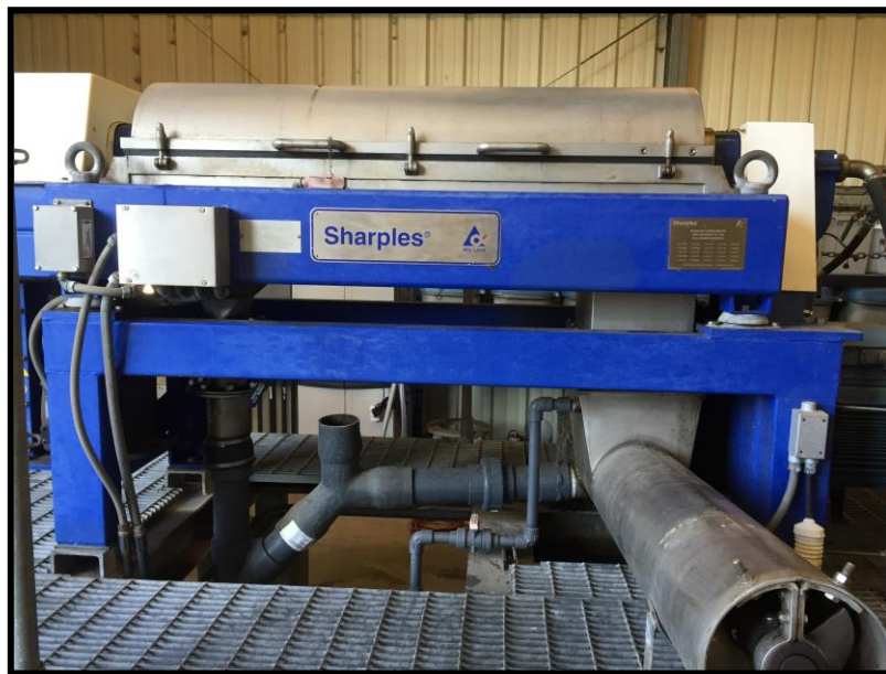
Centrifuge Unit at Rancho Santa FE WRF
