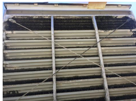
Corrosion of Water Cooling Tower Fin
