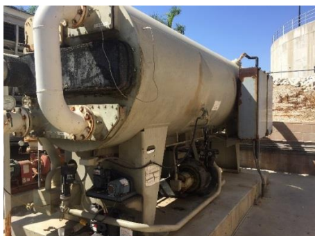
150 Ton Absorption/Condenser Chiller
