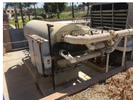
Sealed Vessel (Absorption/Condenser Chiller)
