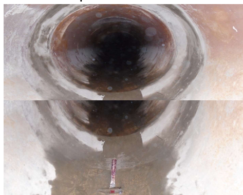
Repaired crack
