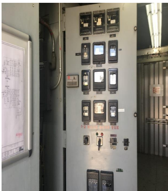
Electromechanical Relays at Freeman
