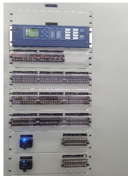
Typical Microprocessor Relays
