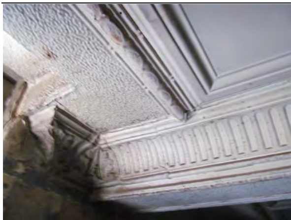
GTL | MHA, March 2015 site recordation photograph; Detail view of interior first floor tin ceiling and cornice trim elements. Proposed for reuse.
