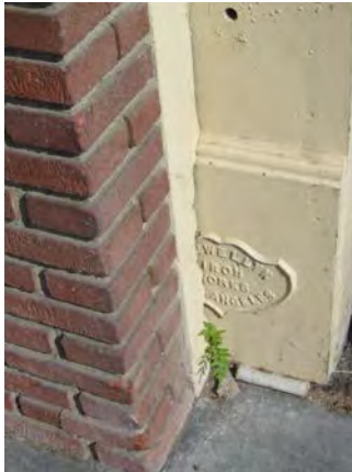
GTL | MHA, March 2015 site recordation photograph; Detail view of exterior west façade, adjacent lot's remaining cast iron column. Station point is approximately 4 feet above grade.
