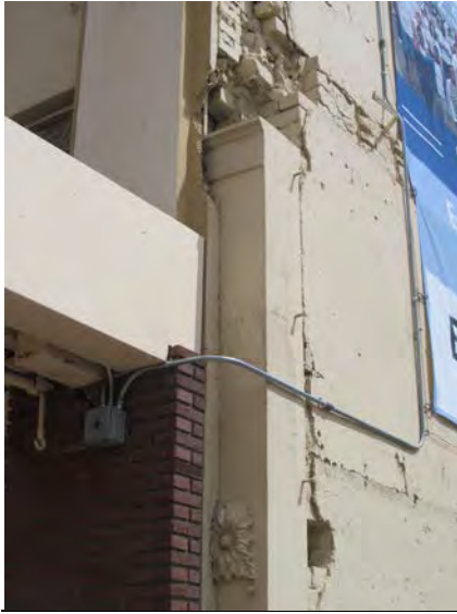
GTL | MHA, March 2015 site recordation photograph; Detail view of exterior west façade, Station Point approximately six feet above the façade, and showing the southwest corner in detail along with the residual cast iron post column proposed to be incorporated in the proposed design.
