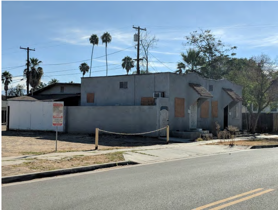
West and south elevation, view looking northeast
