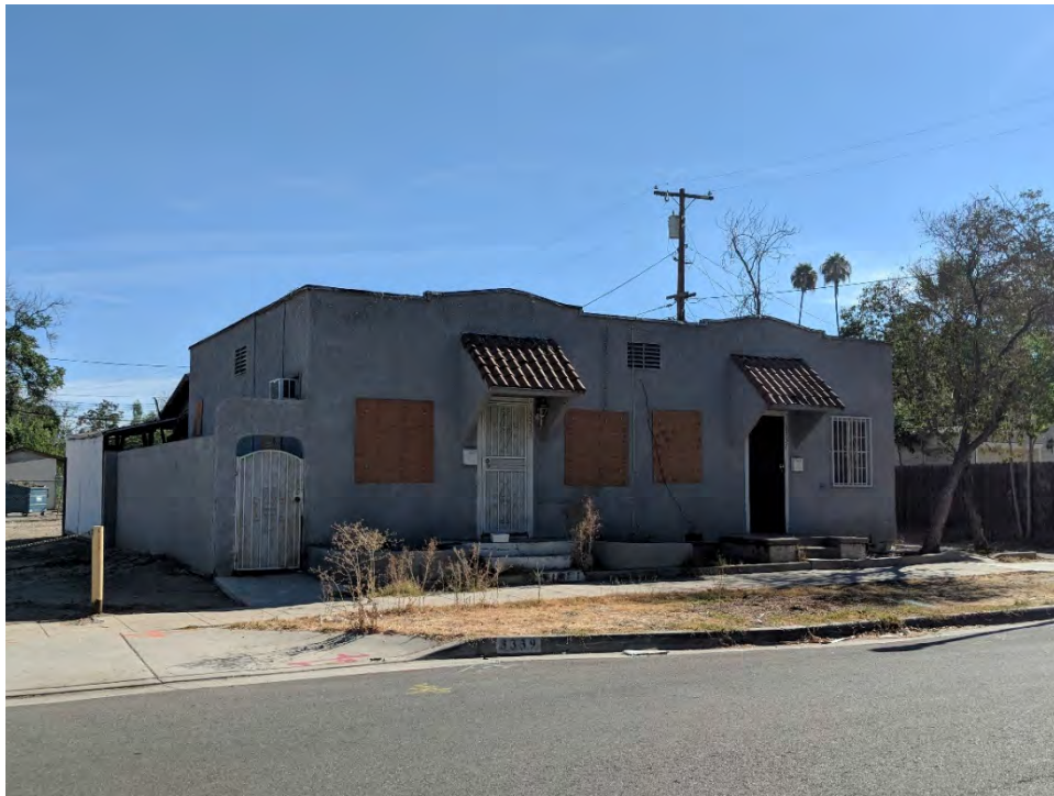
Façade, view looking northeast
