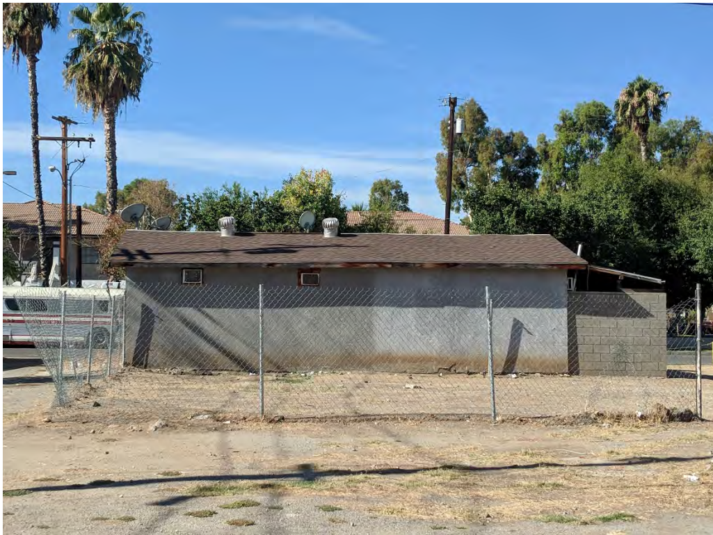
North elevation, view looking southwest
