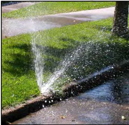
Properly installed swing joints can protect irrigation head breakage that results in high volume run off.
