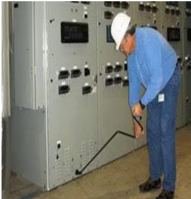
Manual Racking of Circuit Breaker
