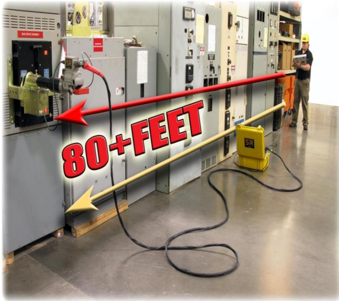
Circuit Breaker Remote Racking
