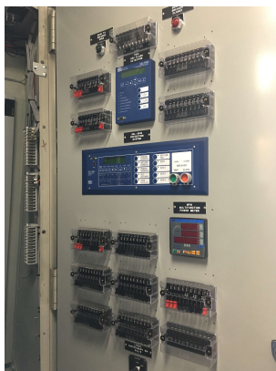
Substation Relay and Equipment Replacements
