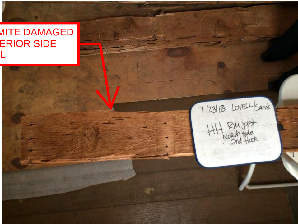
PHOTO 6: NORTH ELEVATION – DAMAGED RIM JOIST
