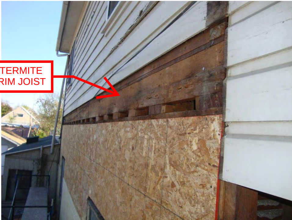
PHOTO 4: NORTH ELEVATION – 2ND FLOOR RIM JOIST
