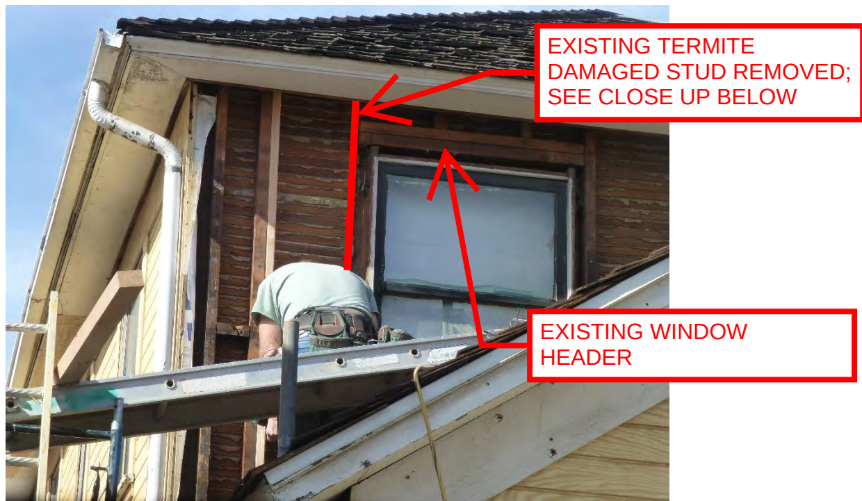
PHOTO 2: EAST ELEVATION – SECOND FLOOR
