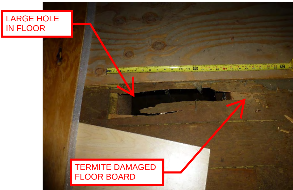
PHOTO 10: DINING ROOM – HOLE IN FLOOR BOARD
