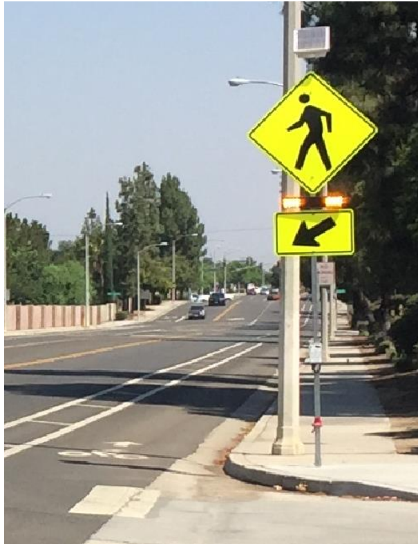
Figure 1: Recently installed RRFB system at Cole Ave & Citrus Grove Rd
