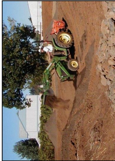
*Soil amendments can be homogeneously incorporated to the recommended soil depth by hand or by equipment, whichever is appropriate for the given project.*
