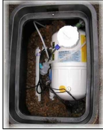
*A fertigation device can be used to provide a liquid fertilizer through irrigation lines*
