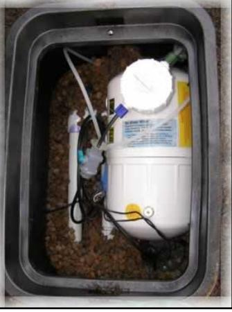
*A fertilization device can be used to provide a liquid fertilizer through irrigation lines*
