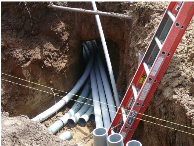
Trench and Conduit Installations
