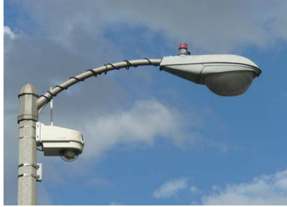
Street Lights with cameras attached
