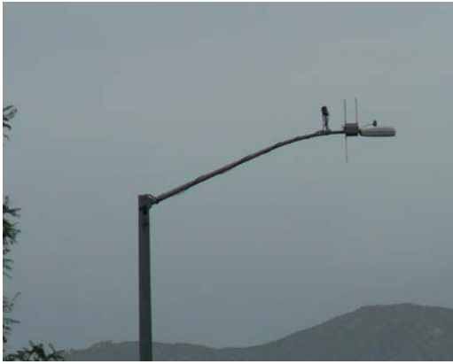
Street Lights with cameras attached
