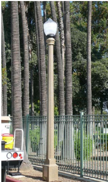
Approved replica standard and luminaire for the Downtown and Wood Streets replacement
