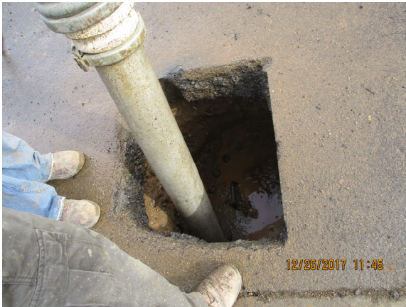
Typical Utility Pothole
