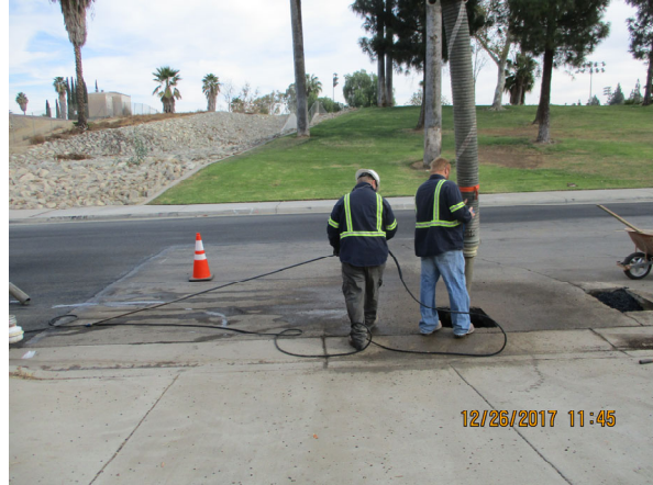
Typical Setup for Identifying Underground Utilities
