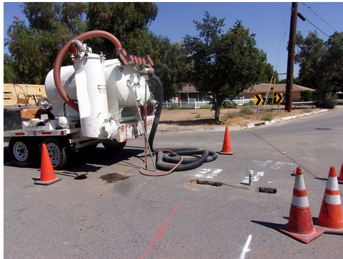
Typical Setup for a Vacuum Excavator
